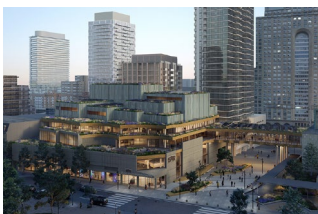
St. Lawrence Centre for the Arts, Toronto, Canada
